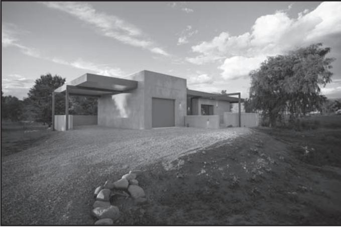
Figure 15. Interesting aesthetic details draw the eye, but don't drag down the building's performance. "If you notice on the steel structures at the Ulibarri's, they are all independent structures from the home's envelope, meaning no risk of thermal bridging," notes Stanford. Photo courtesy Jonah Stanford and NEEDBASED, Inc.
