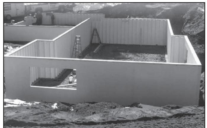
Figure 11. Epitome quality foundation walls, by Composite Panel Systems, LLC, utilize fiberglass and composite technology to create a higher performance, strong, and resilient foundation wall system. Each 24’ Epitome Quality Foundation Wall section withstands greater than 500,000 pounds of downforce providing a max allowable load of 8900 PLF. Photo courtesy Composite Panel Systems, LLC, Fiber-Tech Industries, Inc., and Ashland Performance Materials.
