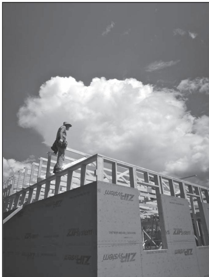
Figure 14. Jonah Stanford used ZIP System® panels to ensure airtightness in the home's roof and shell. Photo courtesy Jonah Stanford and NEEDBASED, Inc.
