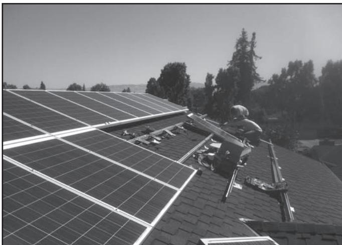
Figure 7. Installation shot of Cottle's solar photovoltaic (PV) panels. Photo courtesy One Sky Homes.
